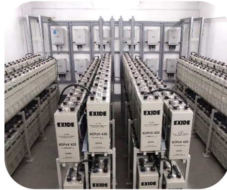
Exide CESC BESS Gel Based VRLA
