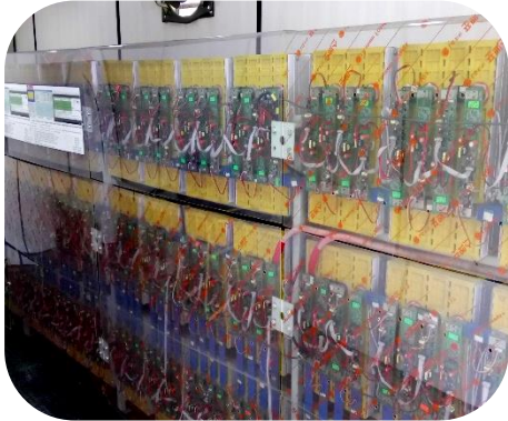
Hosur ESS Lithium Ion
