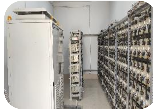
Lead Acid Battery Banks at a newly commissioned microgrid project in Kolkata
