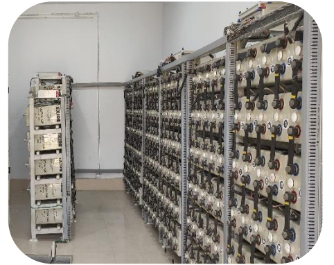
CESC Microgrid Gel Based VRLA
