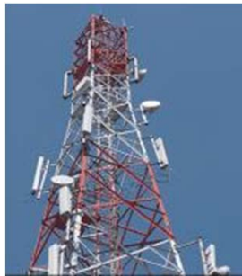
BTS-Base Transceiver Station
