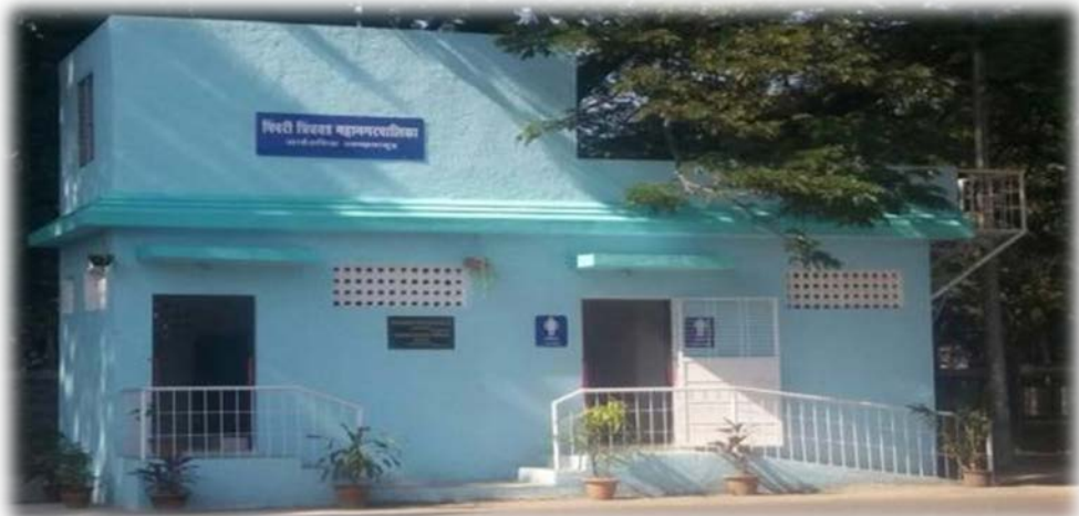
Public Sanitation facility built at Chinchwad
