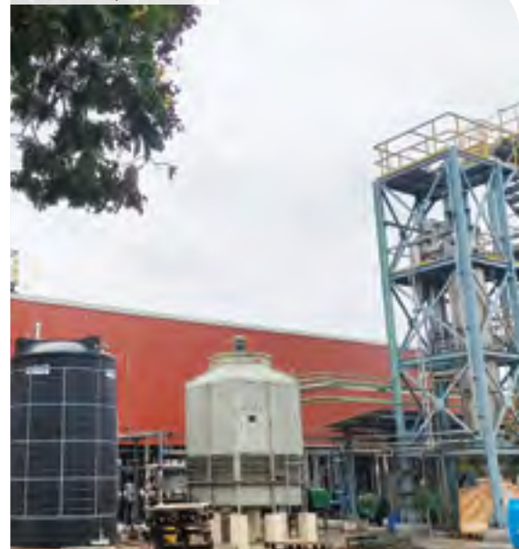
ZLD at Hosur plant
