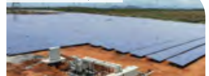
Off-site Exide solar panels
