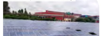
On-site solar panels at Exide facility
